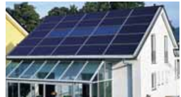
Complete roof installation
