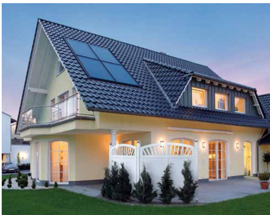
Premium in-roof installation
