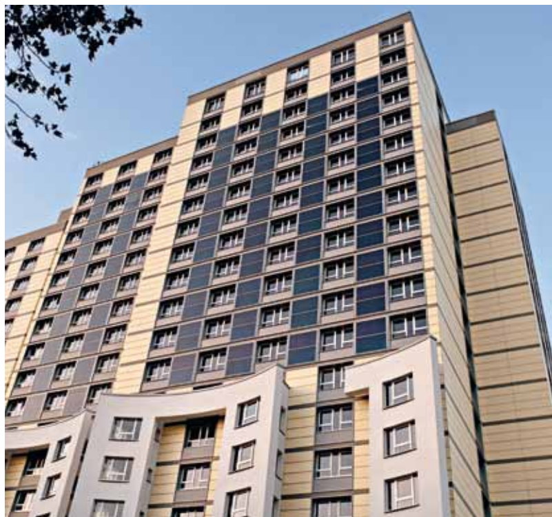
Large thermal system in the façade of an apartment block
