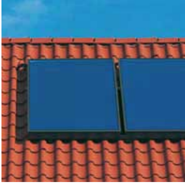
On-roof installation
